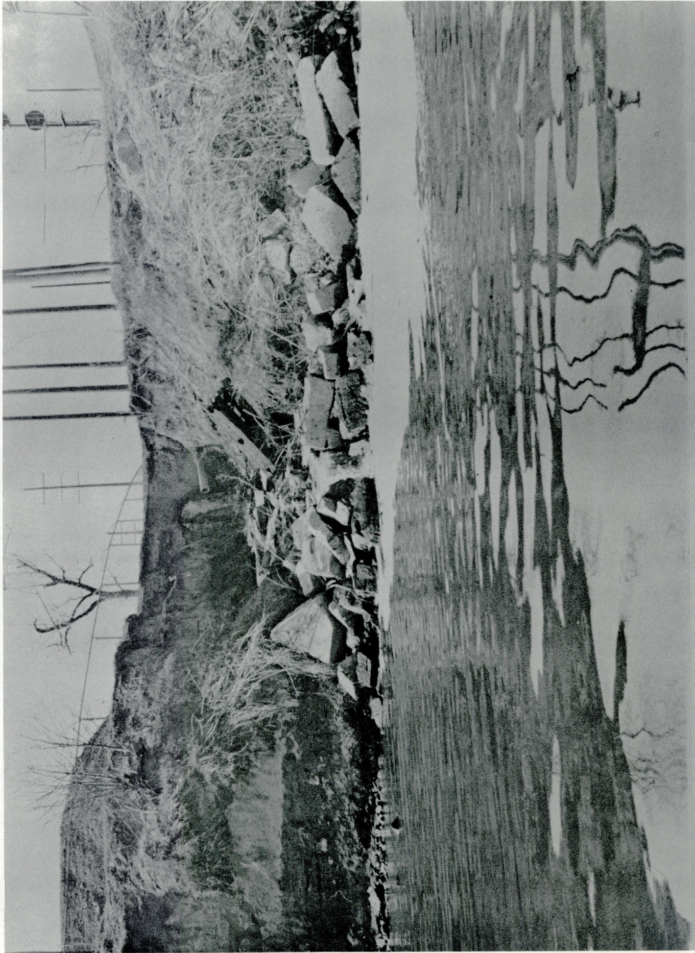
Sewer outlet along area of Stickney Sewage Treatment Works sludge lagoons. Discharging waste water believed to be either overflow or underdrainage from lagoons.
