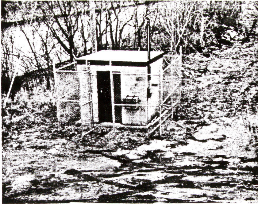
AVM shelter 8 X 8 concrete block constructed Mar 1984
