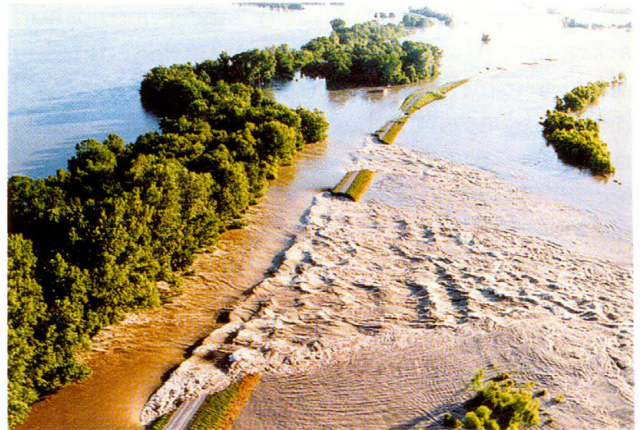
Breached levee along the Mississippi River. (Photograph courtesy of the St. Louis Post Dispatch.)
