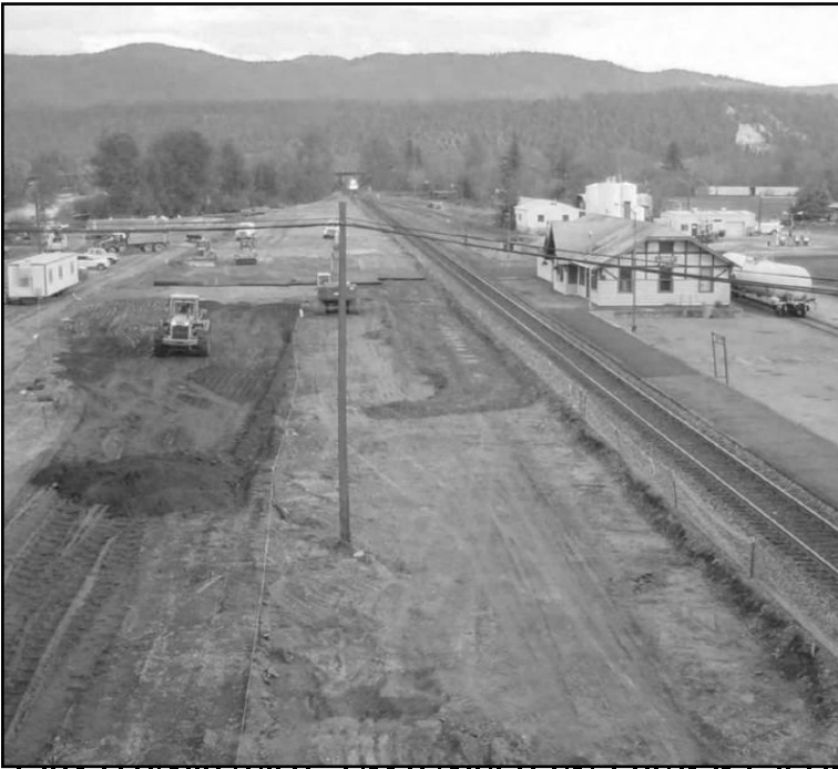
4-ER-914 (excavation); 4-ER-915 (capping and backfill).
