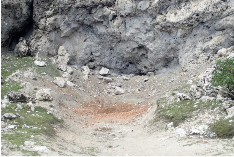
Photo 8. OD unit close-up (2-3 feet deep)
