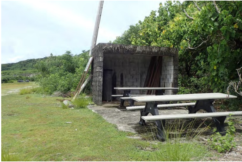
Photo 4. Cement/personnel bunker (looking east)
