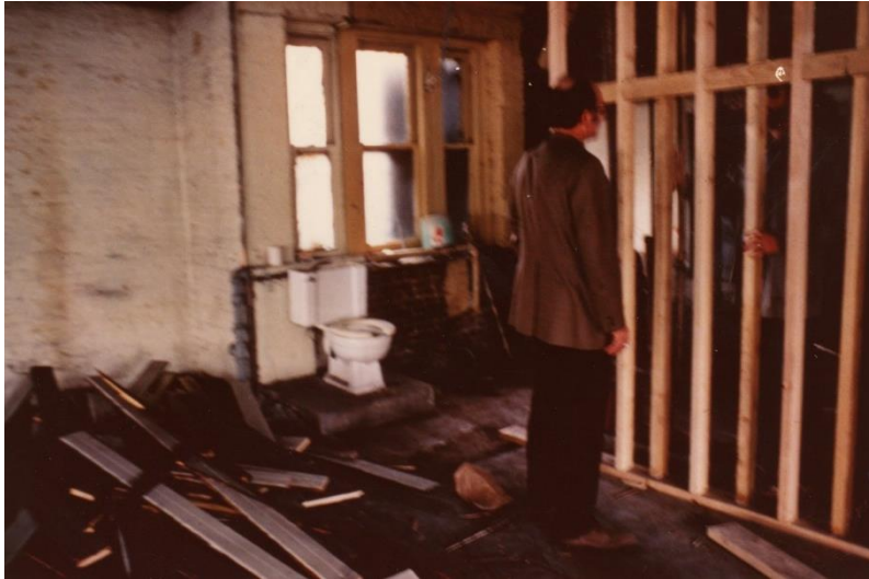
Putting up a new loft wall, in SoHo Memory Project (n.d.), https://sohomemory.org/loft-renovation-first-wall-n-d/ .
