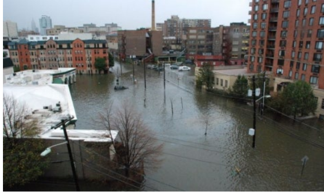
Figure 14: Hoboken Underwater due to Superstorm Sandy Storm Surge 285
