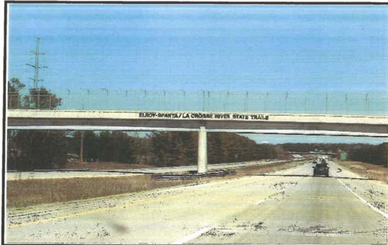
FIGURE 2: Pedestrian overpass for Elroy-Sparta/La Crosse River State Trails.
