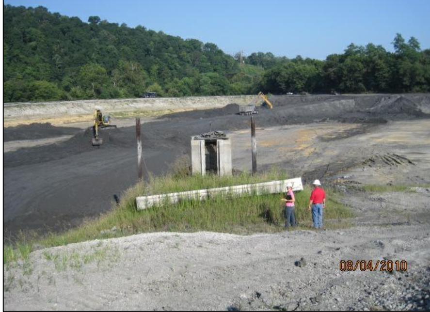
4-1 FROM SOUTHEAST DIKE LOOKING NORTHWEST AT INACTIVE OUTLET STRUCTURE AND POND INTERIOR
