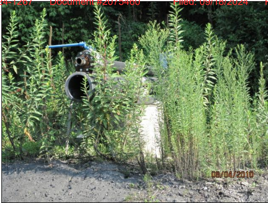
4-9 INLET STRUCTURE FROM PLANT ON NORTH DIKE
