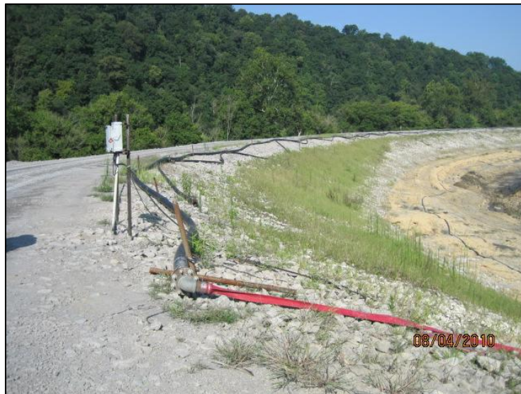
LOOKING WEST FROM SOUTH DIKE AT CREST, UPSTREAM SLOPES AND HDPE PIPES USED TO TRANSPORT CCW TO POND #2
