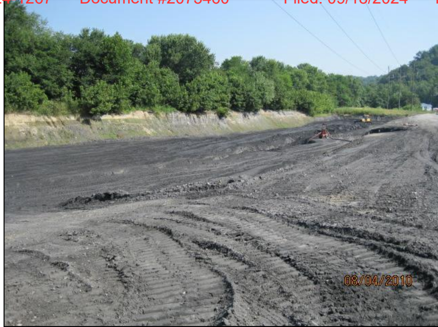
3-1 FROM SOUTH END OF COMMON DIKE LOOKING NORTHWEST
