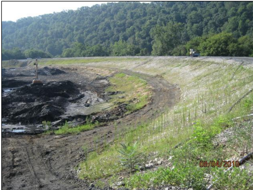
4-10 LOOKING SOUTH FROM NORTH DIKE
