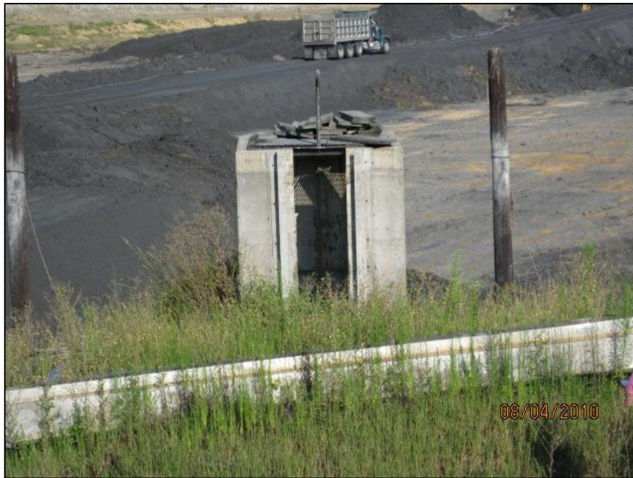
4-2 INACTIVE OUTLET STRUCTURE
