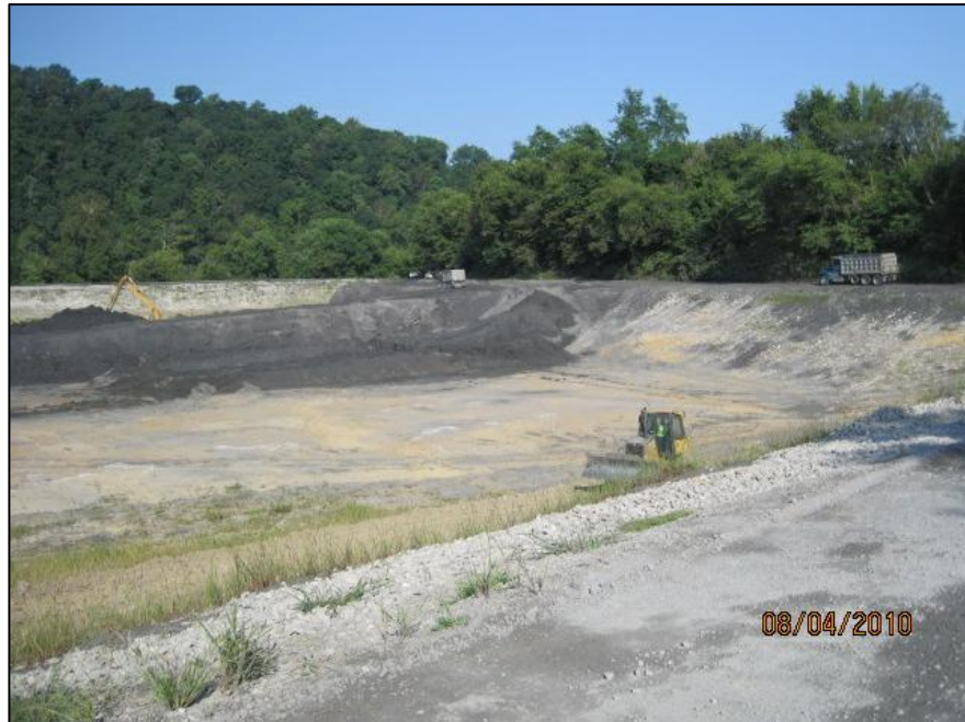
4-8 LOOKING NORTHWEST FROM EASTERN DIKE
