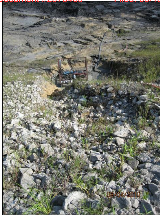
PUMP UTILIZED DURING LOWERING OF PHREATIC SURFACE, EXCAVATED SUMP AND EROSION GULLEYS ON UPSTREAM SLOPE
