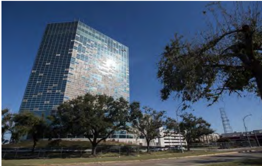
The shuttered Capital One Bank Tower is pictured Thursday, January 13, 2022, in Lake Charles, La.
