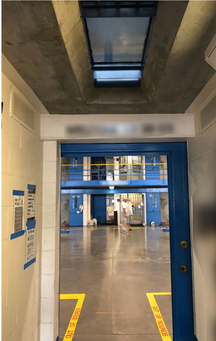
Photo 4. Prison section entryway; solid prison cell doors shown. (Photo taken by OIG staff on October 8, 2020, at California State Prison, Corcoran.)
