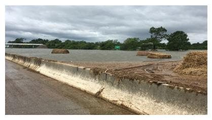
24. Likewise, in September 2019, TxDOT's median barrier/dam along IH-10 blocked rainfall runoff from overtopping the roadway during and after Tropical Storm Imelda. During Imelda eastbound traffic lanes remained open and conferred a benefit to the public at
