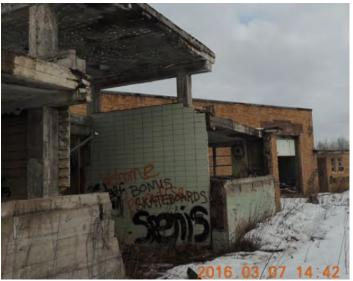
The property was subject to a significant amount of trespassing, looting, graffiti, and fire and water damage after it was abandoned prior to forfeiture; and the building's roof had failed and was open to the elements for many years. Large quantities of
