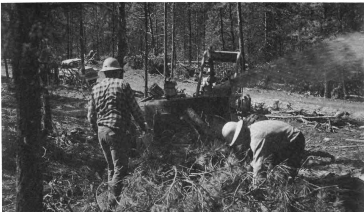
Figure 5.—Mechanical Chipper Disposing of Fuel Debris in the Ocheco National Forest, Oregon, 1961—U.S. Forest Service photo.
