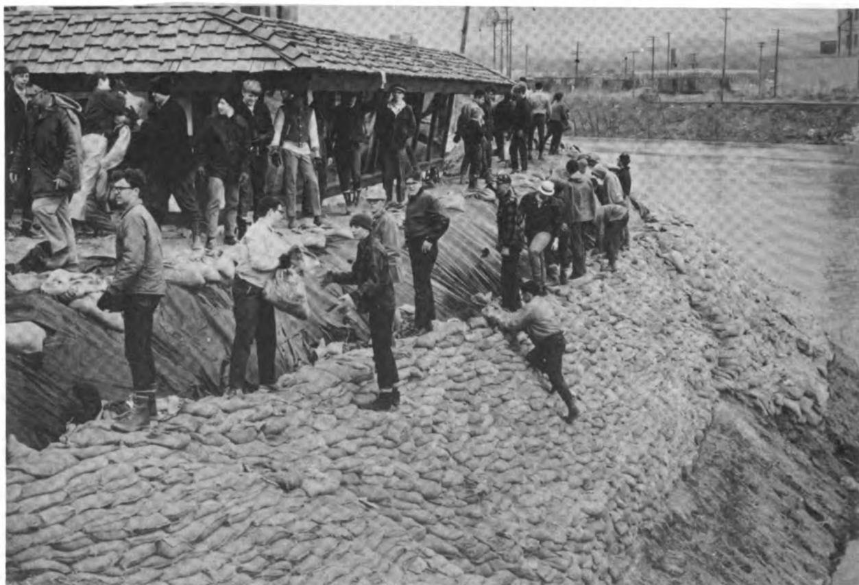
Figure 6.—Operation Foresight 1969. Right: women of North Mankato join the fight and fill sandbags for protective works—OEP photo. Below: teenagers and older men of North Mankato anchor sheets of polyethylene with sandbags to prevent current scouring of the temporary levee—photo from National Geographic , October 1969 (pp. 580-581), Photographer Thomas Defeo, (c) 1969 National Geographic Society, reprinted with permission.
