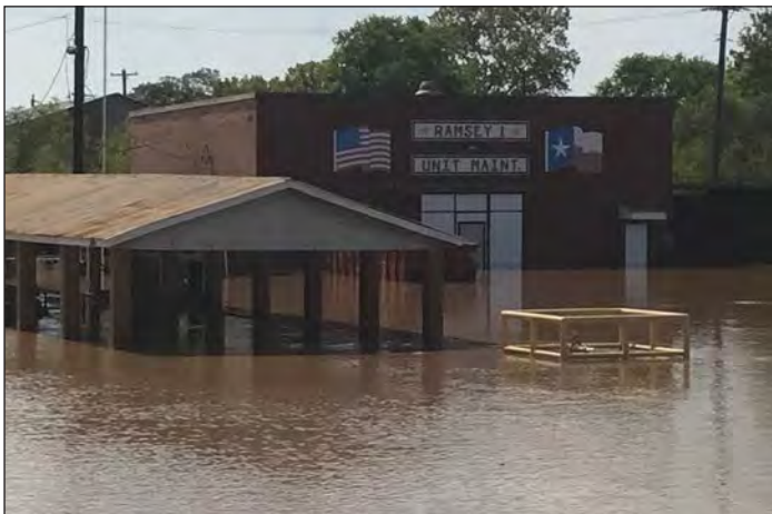
The maintenance building at the Ramsey Unit in Rosharon, Texas during flooding caused by Hurricane Harvey.
